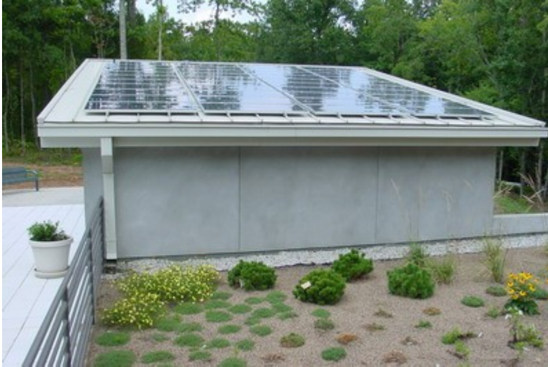
Figure 2: Solar Array, Sweetwater Creek Visitor Center, from southface.org
